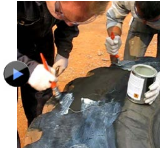
Video 7.1 Application of MetaLine 910 Rubber Primer
